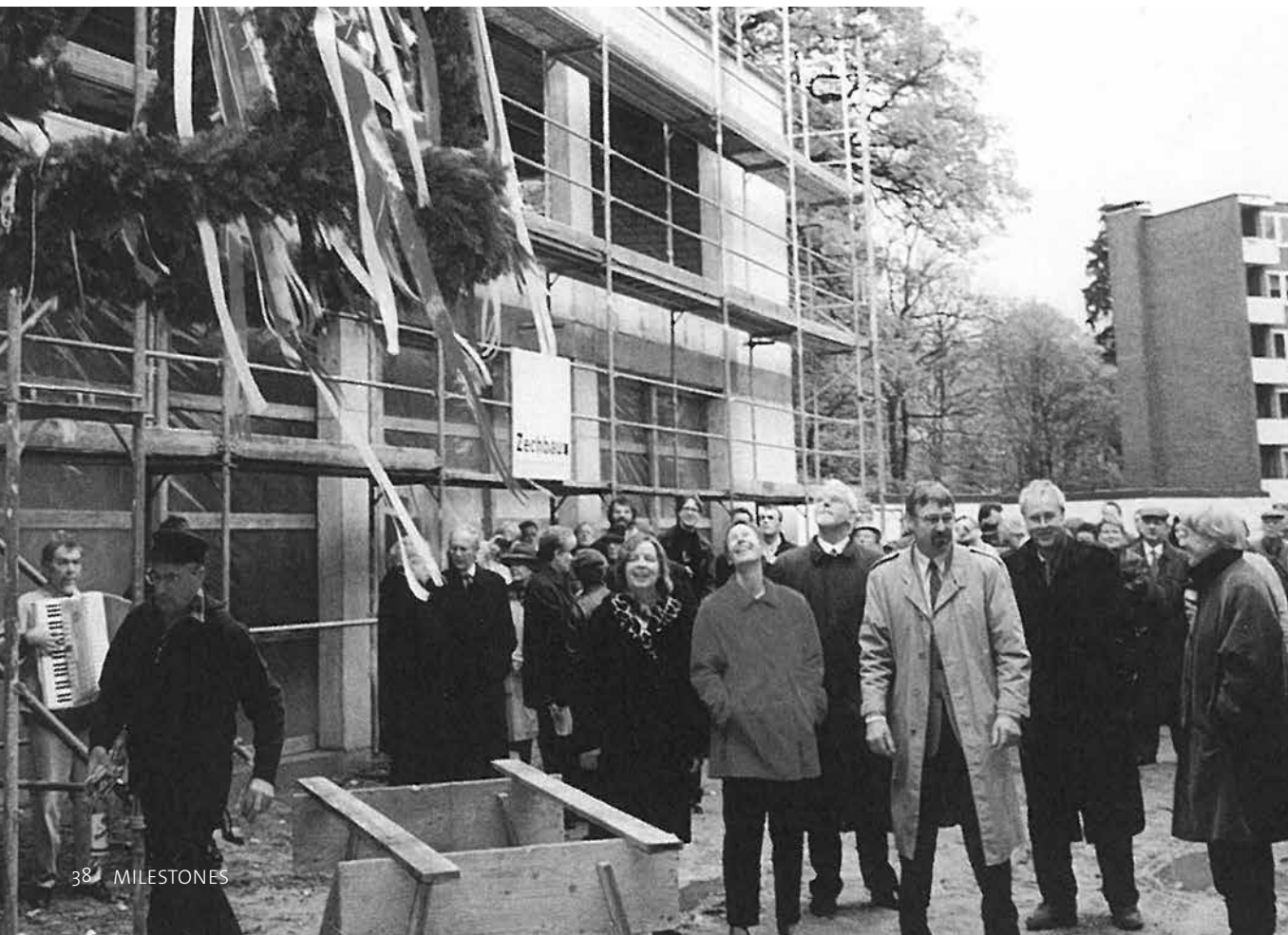
Placement of the topping-out crown on top of the shell construction of the Hanse-Wissenschaftskolleg on 7 November 1997.
